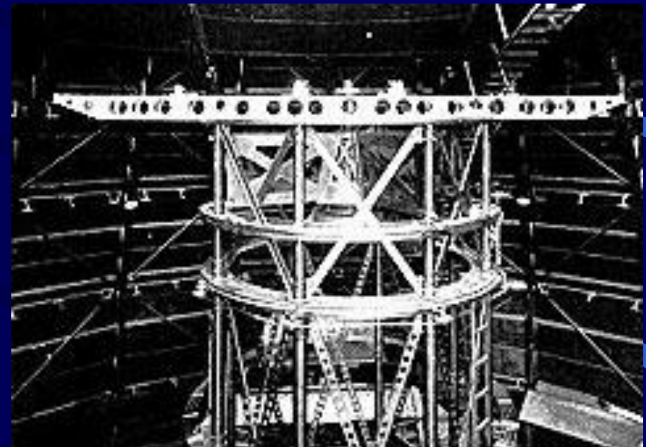
The 20-foot beam on top of the 100-inch Hooker Telescope on Mt. Wilson in Southern California.
